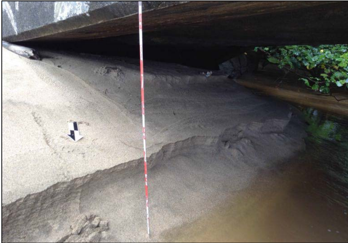
Figure 64. SIHP # 50-30-03-2298, the Waikoko Stream Bridge, underneath profile view to south of the 1912 portion of the bridge undermined by the 1946 tsunami
