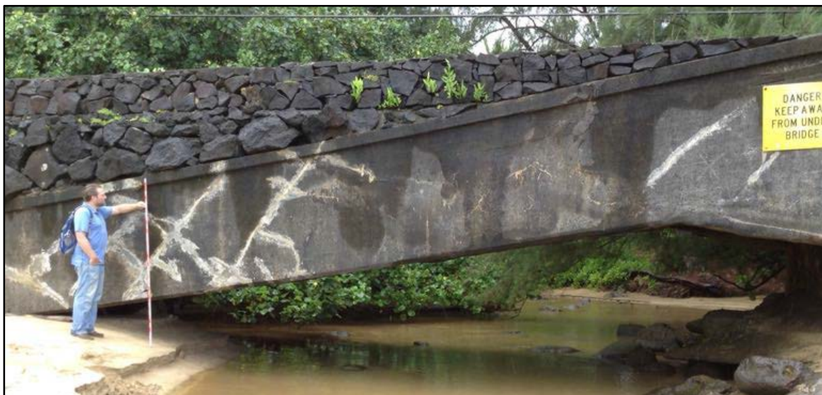
Figure 65. SIHP # 50-30-03-2298, the Waikoko Stream Bridge, profile view to southwest; note the 1912 portion of the bridge undermined by the 1946 tsunami, with portions of the overlying basalt boulder and mortar repair
