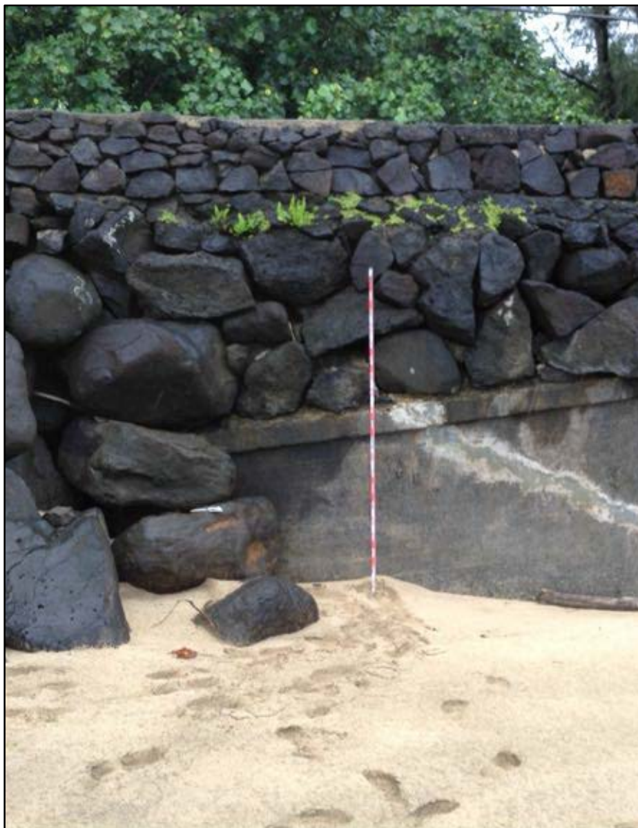
Figure 66. SIHP # 50-30-03-2298, the Waikoko Stream Bridge, profile view to southwest; note the 1912 portion of the bridge undermined by the 1946 tsunami, with portions of the basalt base coarse and overlying basalt boulder and mortar repair
