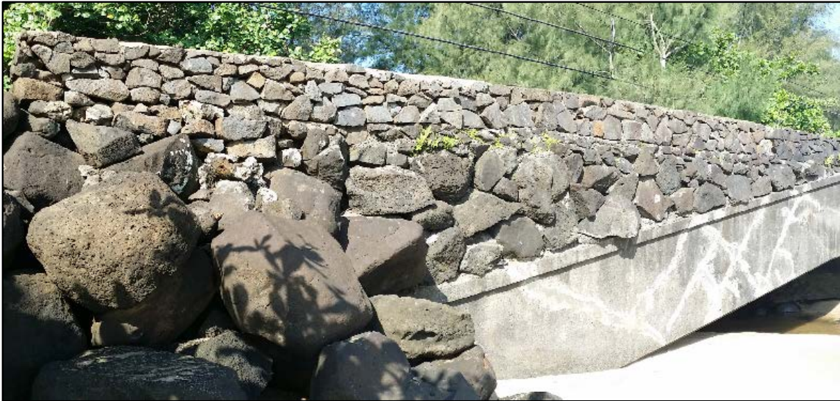
Figure 60. SIHP # 50-30-03-2298, the Waikoko Stream Bridge, general view to west of the bridge's makai face; note approximately eight courses of basalt boulders mortared on top of the concrete portion of the bridge damaged in the 1946 tsunami
