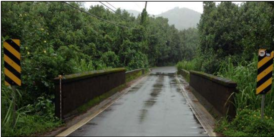
Figure 54. SIHP # 50-30-03-2297, the Waipā Stream Bridge, view to north; note the 1912-built bridge portion in the foreground
