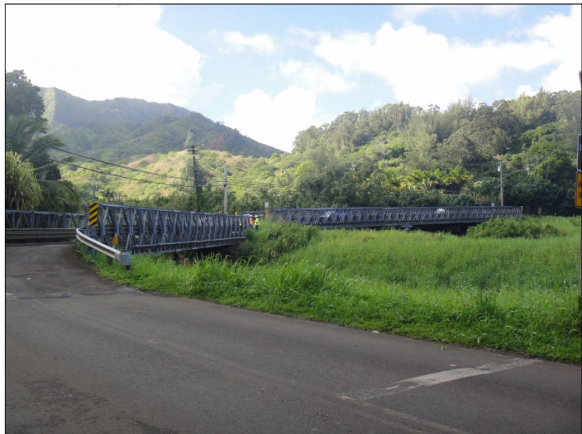
Photo of existing Bridges 2 and 3 and how they operate as one bridge
