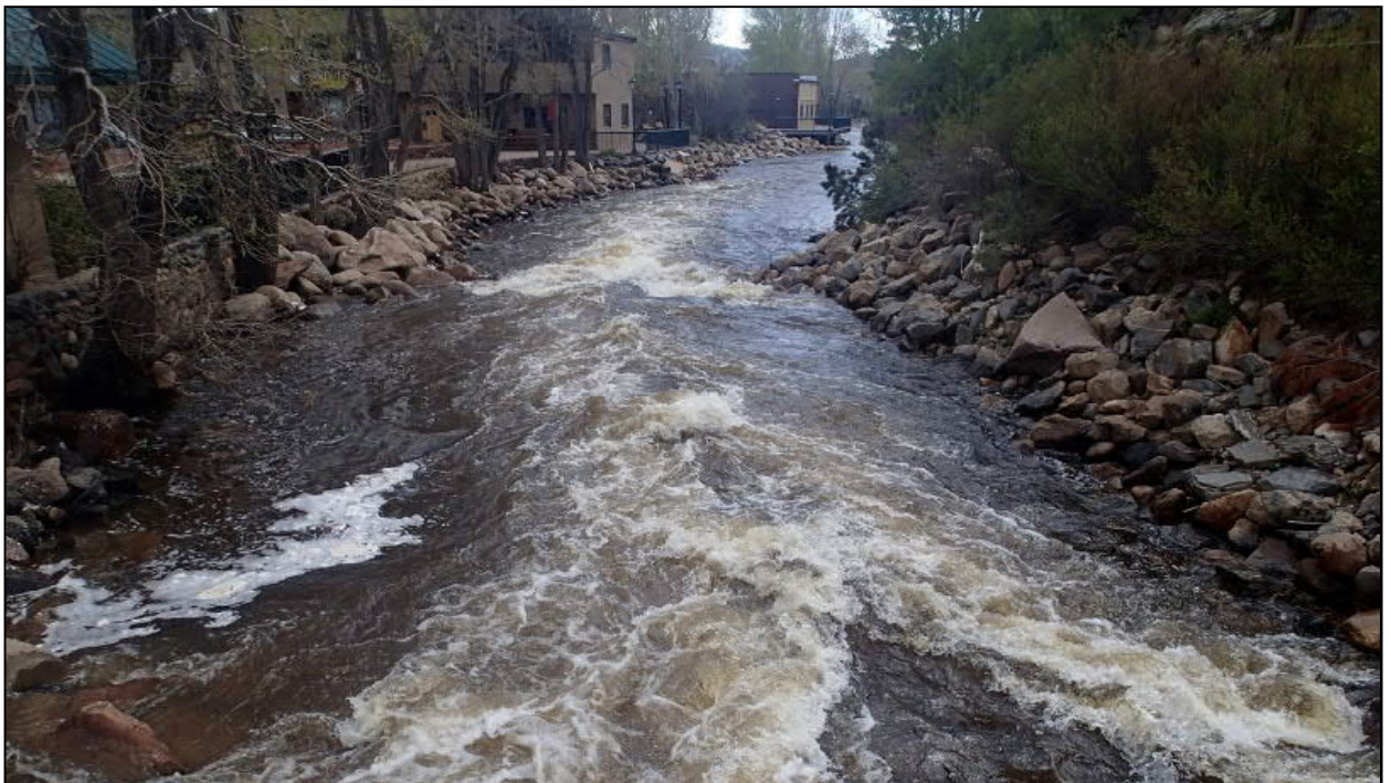
Figure 3.15-14: View of the Big Thompson River (facing east) Downstream of Riverside Drive Bridge
