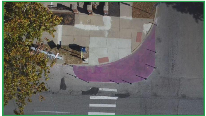
A drone image of a curb extension at the intersection of Linn Street and Chestnut Street in Cincinnati. Source: Christian Hauser.
