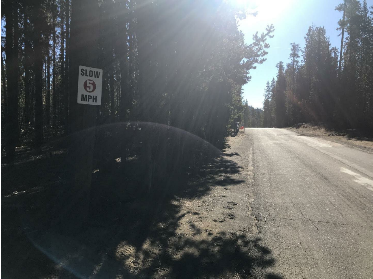
Figure 51 - Non-MUTCD Compliant Sign east of Elk Lake Intersection, Elk Lake Lodge Road, Looking East
