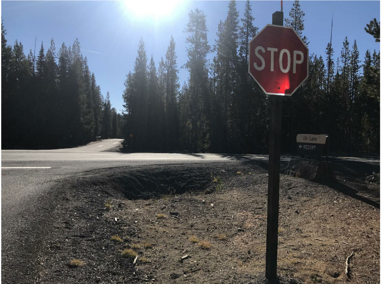
Figure 45 - Stop Sign on West Quadrant of Elk Lake Intersection, Elk Lake Trailhead Road, Manufactured May, 2018, 30" x 30"
