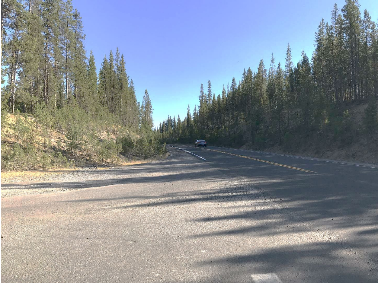
Figure 56 - Lava Lake Rd. Intersection, Limited Sight Distance to South
