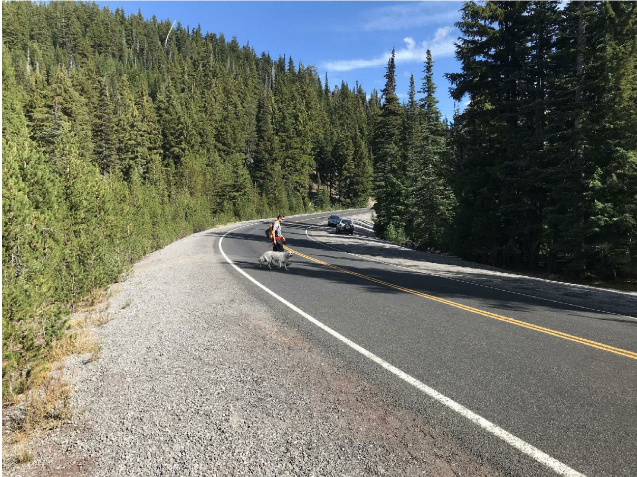
Figure 33 - Pedestrian Crossing near Apex of Curve at Devils Lake
