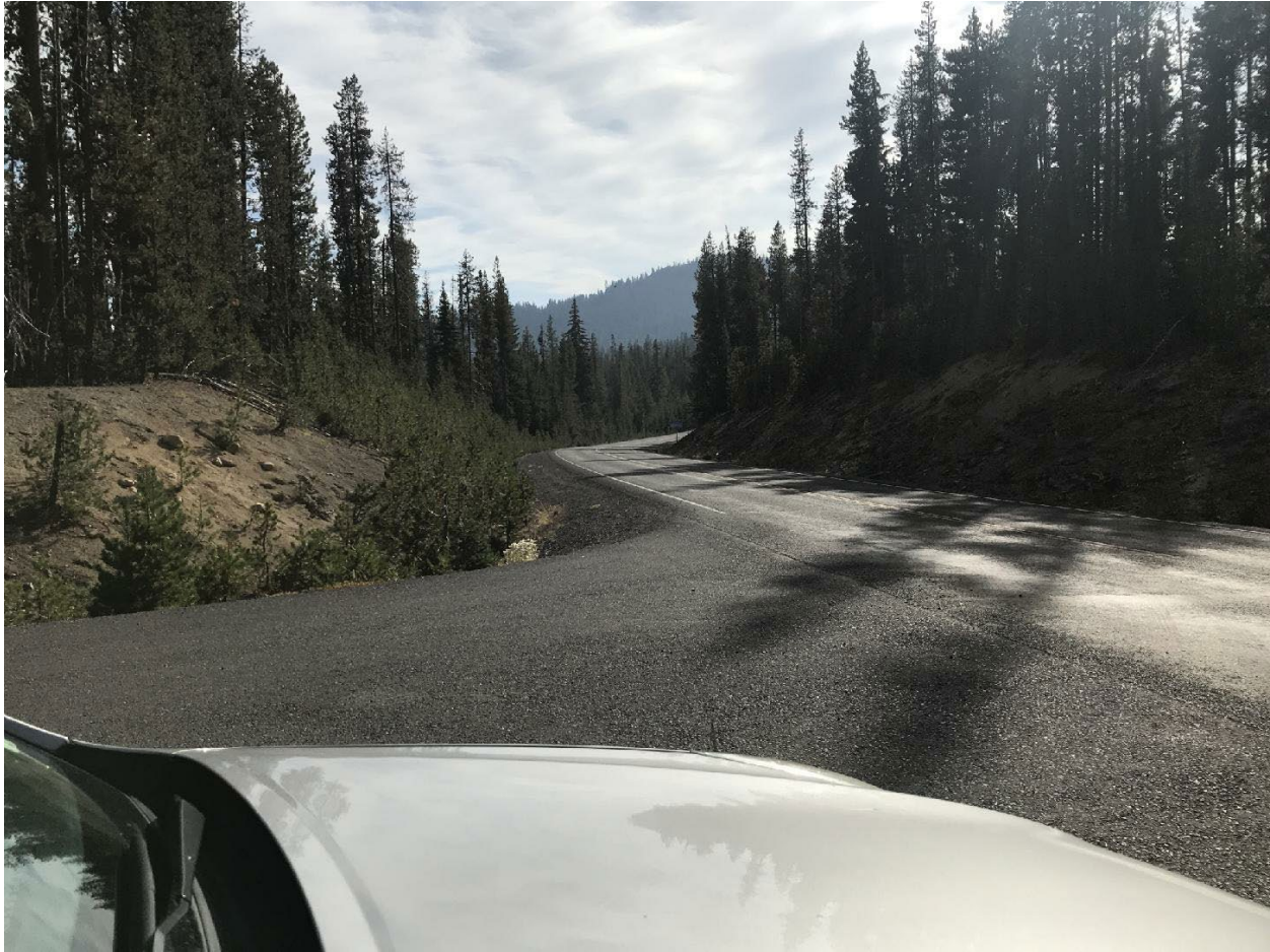
Figure 41 - NF-4625 Intersection - Sight Distance to South
