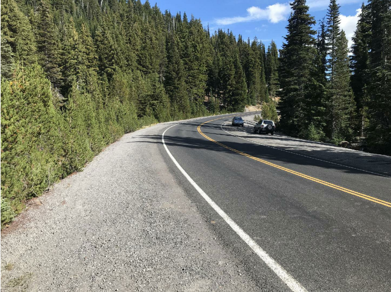
Figure 34 - Devils Lake Trail Crossing, Looking North/East
