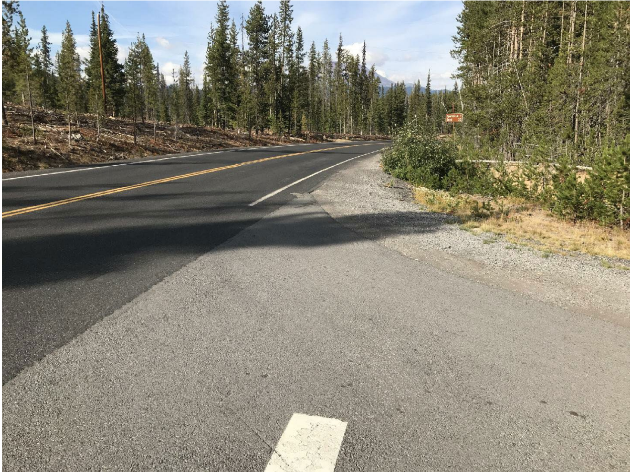
Figure 50 - Intersection Sight Distance at Elk Lake Intersection East Quadrant, Elk Lake Lodge Road, Looking North
