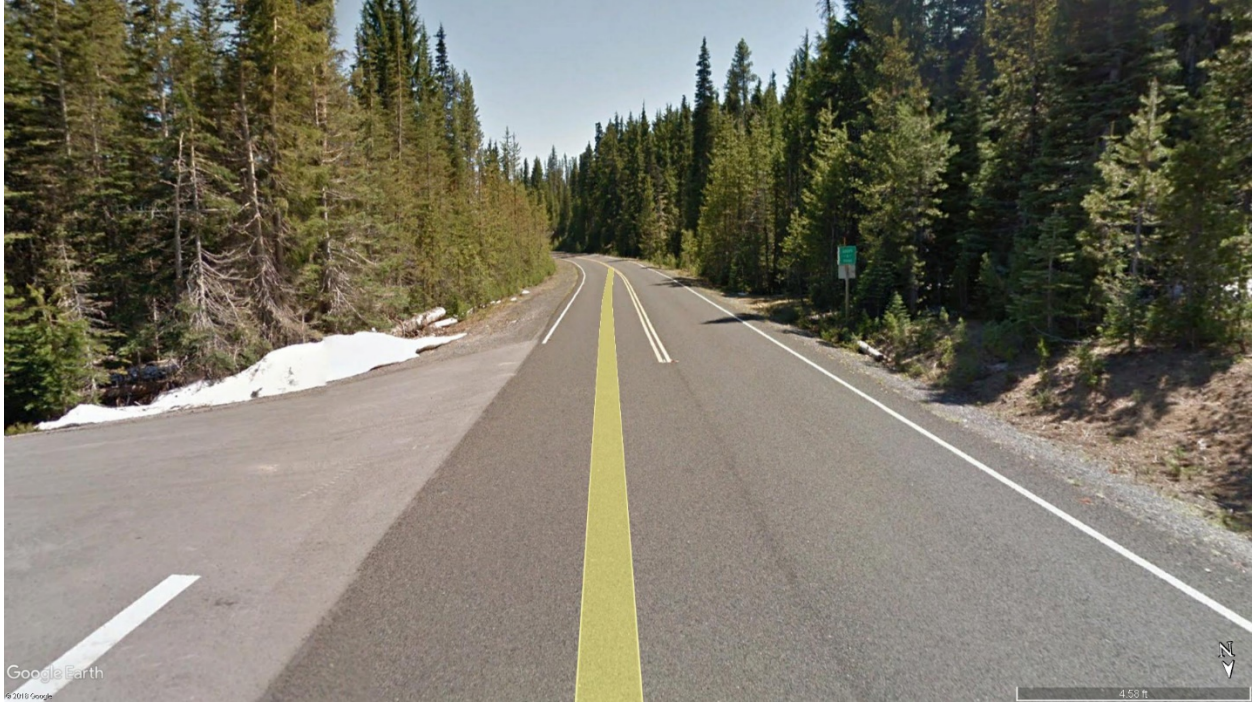
Figure 54 - CLH Intersection with NF-4600 (Point Campground), Looking South
