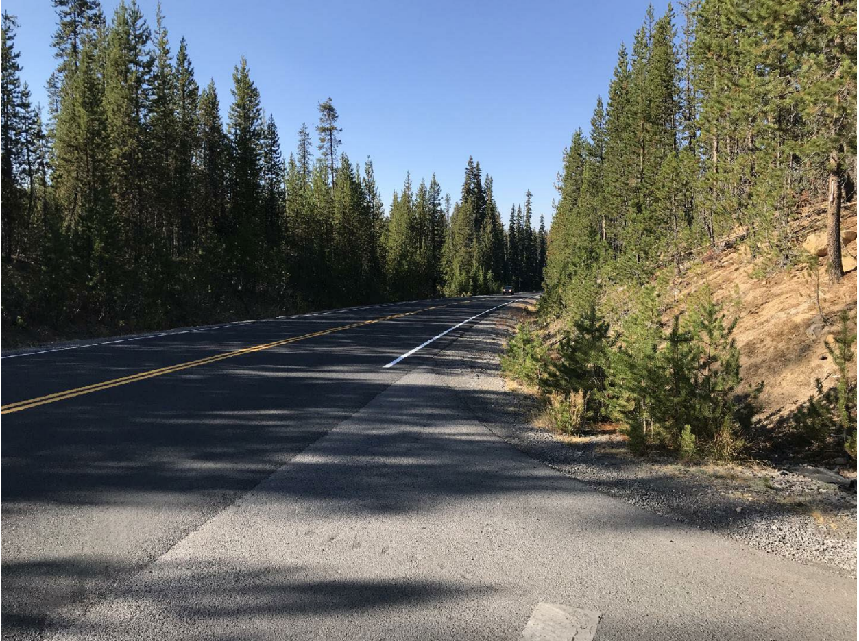
Figure 55 - Lava Lake Rd. Intersection, Limited Sight Distance to North
