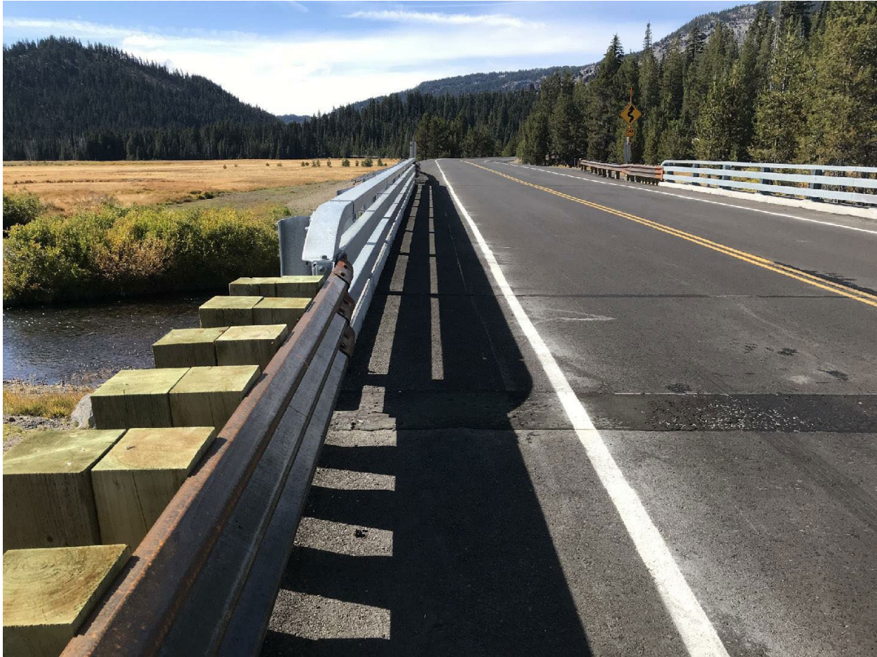
Figure 13 - Recent Bridge Replacement Near Green Lakes Parking Lot
