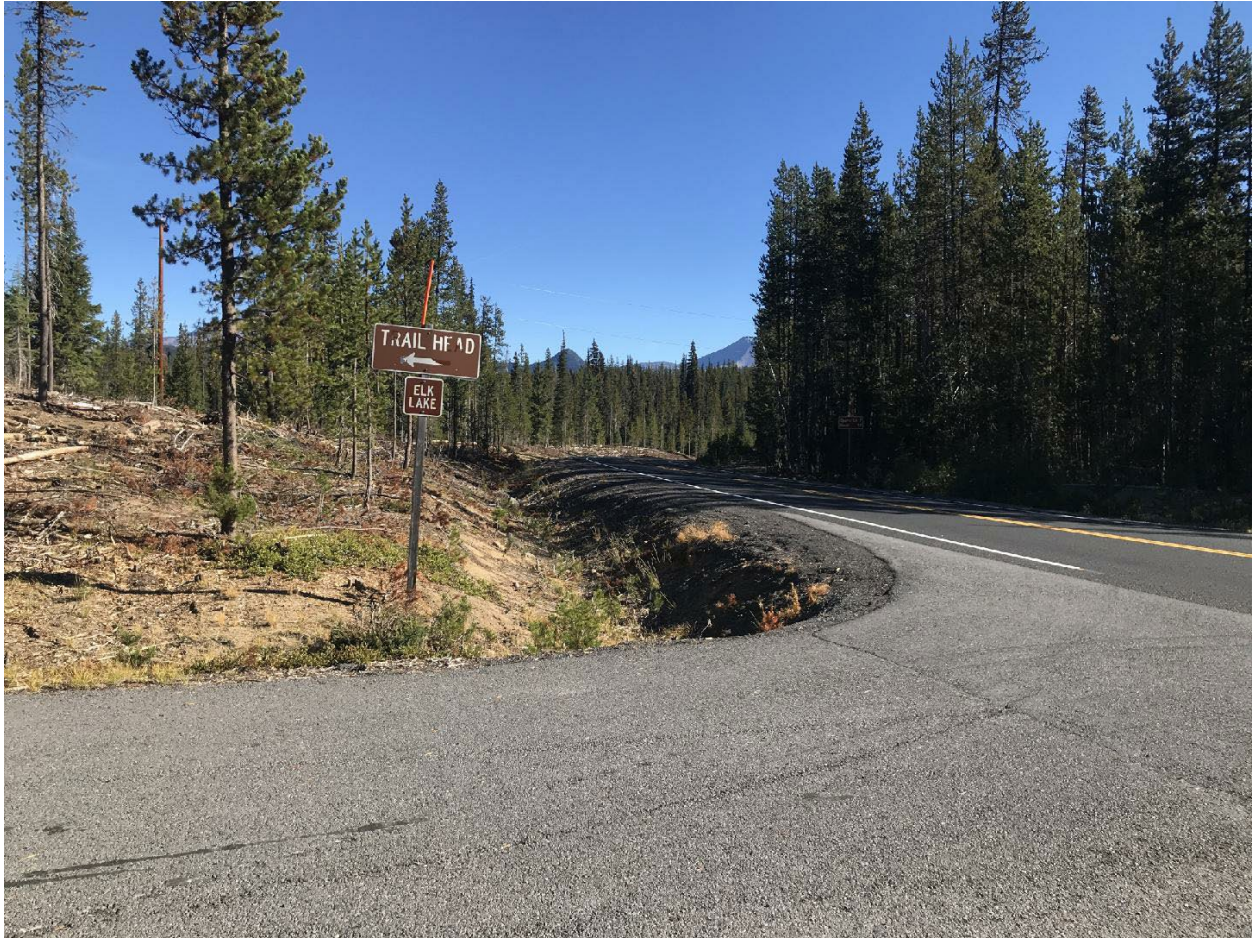
Figure 48 - Guide Sign in Poor Condition, West Quadrant of Elk Lake Intersection, Elk Lake Trailhead Road, Looking North
