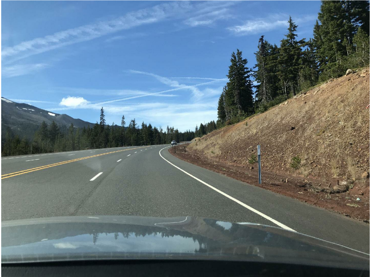
Figure 17 - ODOT Portion of CLH - Route Continuity - Approx. 43°58'57.35"N, 121°37'19.02"W
