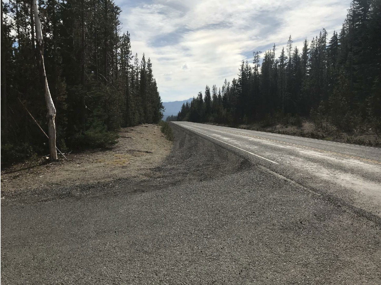
Figure 40 - CLH Intersection with NF-450 (Quinn Meadows), Limited Sight Distance to South
