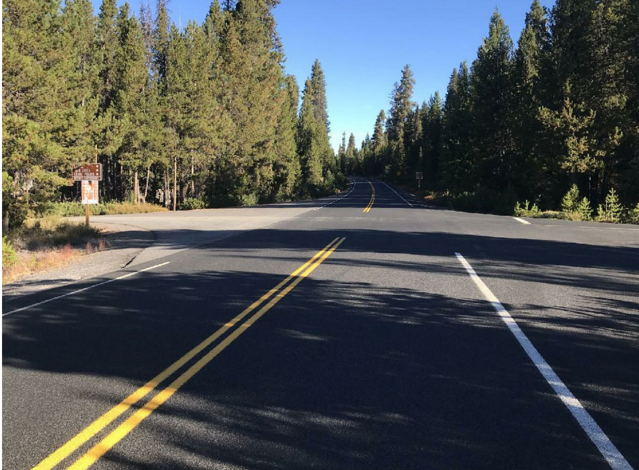
Figure 61 - CLH Intersection with S. Century Dr., South Approach, Looking North
