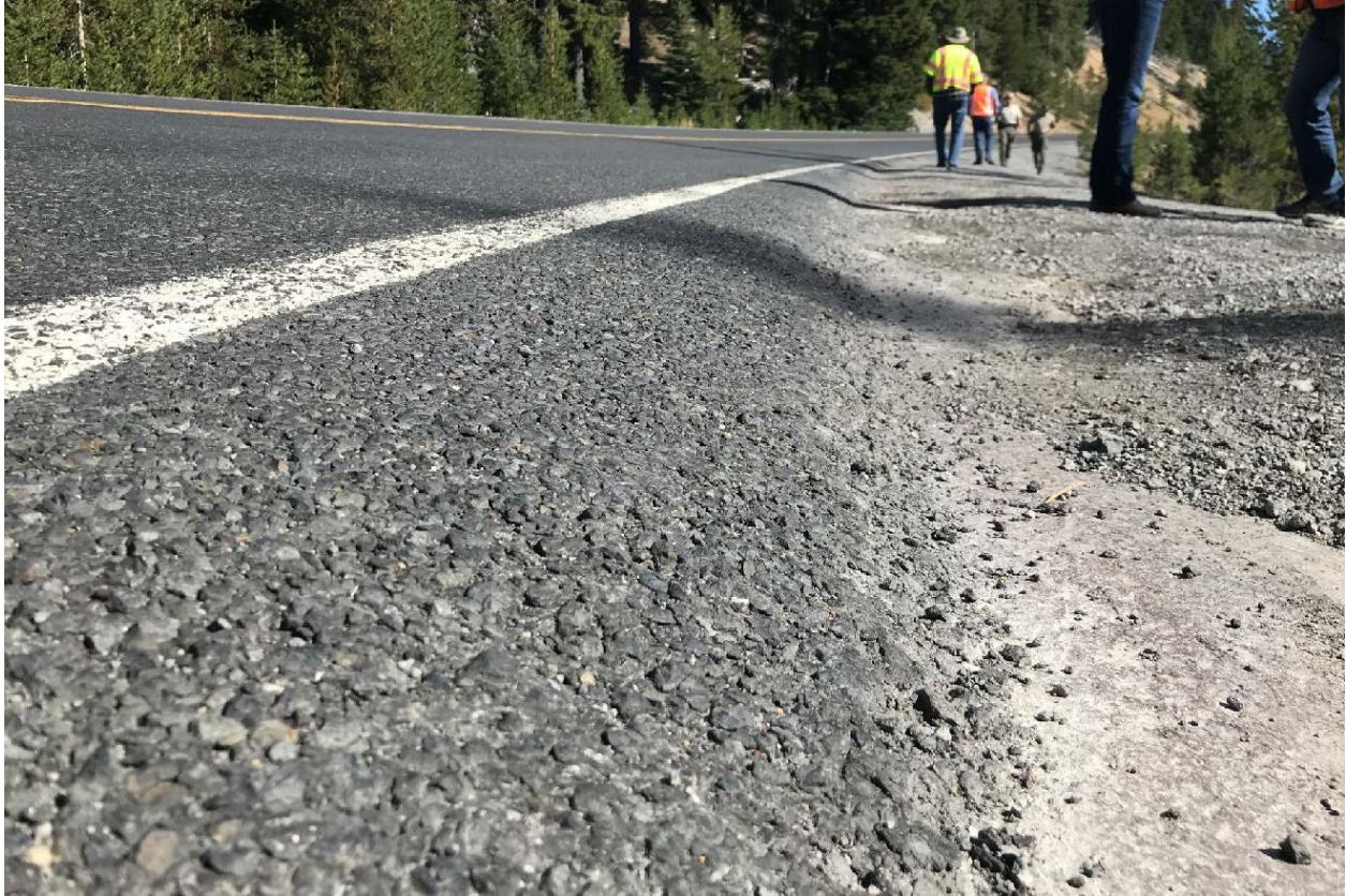
Figure 38 - Pavement Edge Drop-off Near Gravel Turnout at Devils Lake, Approx. 3" in Height
