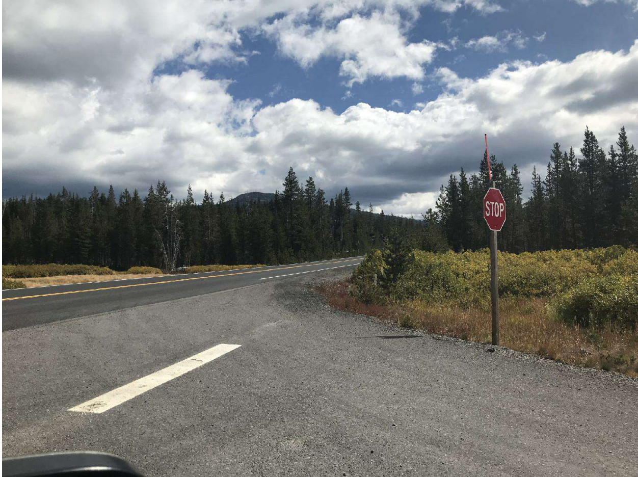
Figure 5 - Todd Lake Intersection, Southwest Quadrant, Looking Southeast
