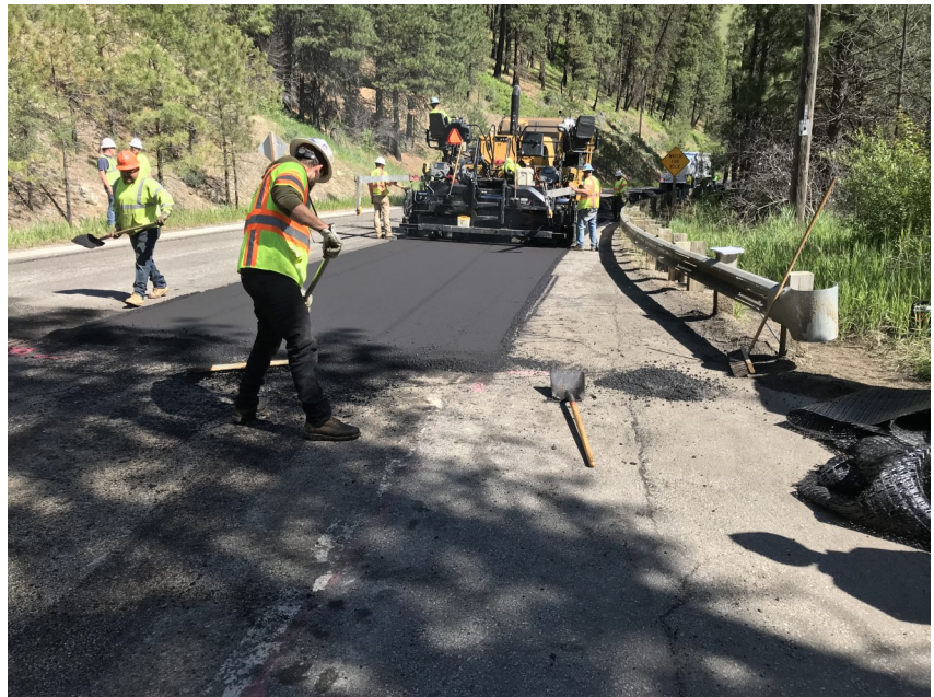
Start of the Paving.
