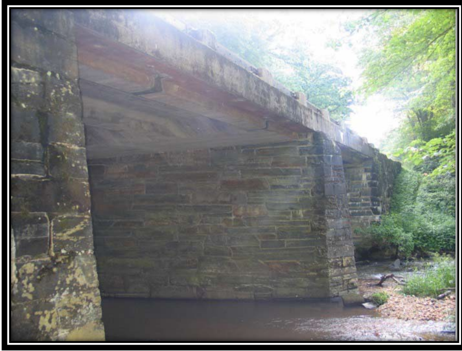
Exhibit 3: Brush Creek Bridge #1, Structure 5140-081P – Side view of bridge degradation
