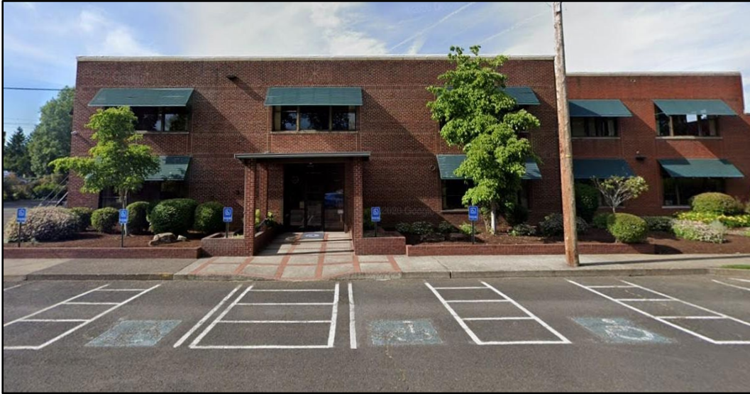
Photo: Front entrance to the WFLHD Main Office Building
