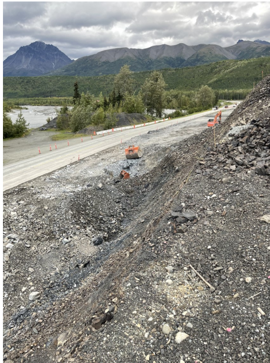
Left: Shot rock excavation adjacent to the Glenn Hwy.
