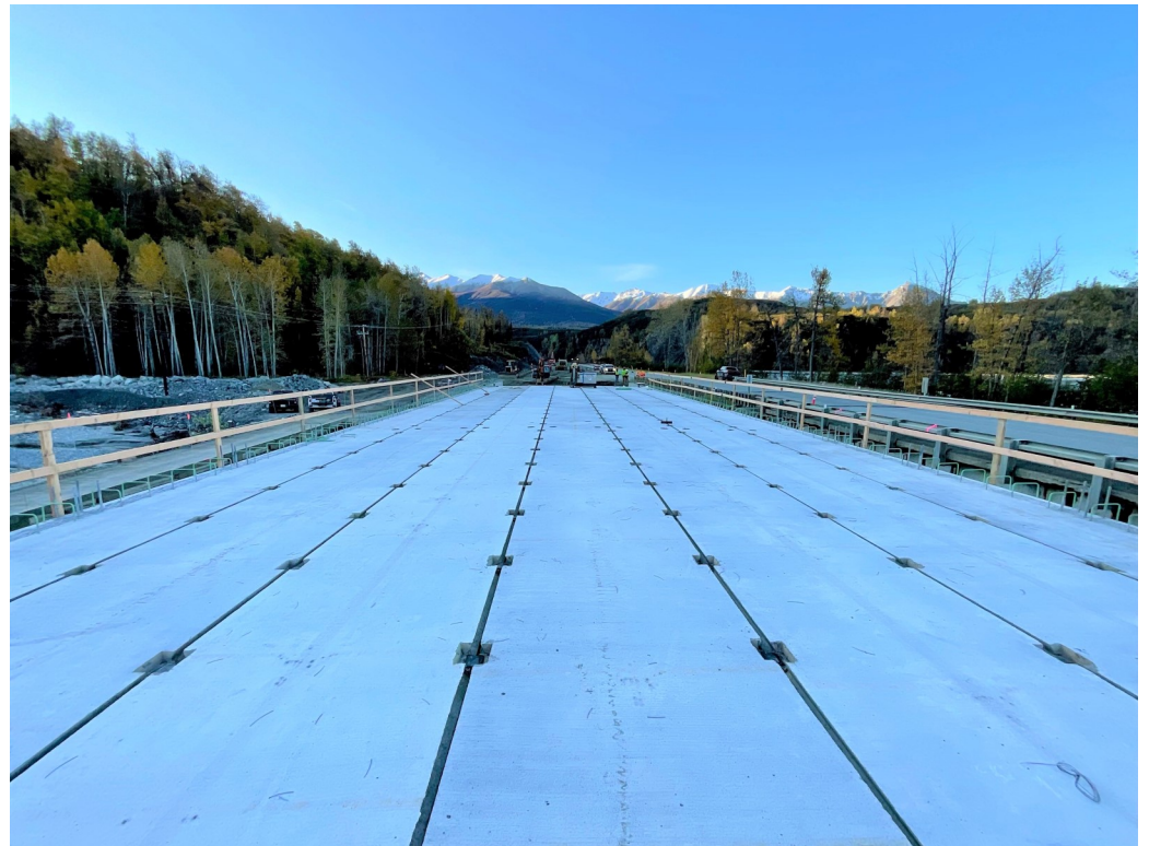
Above: Southbound girders in place.
