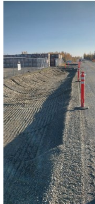
Above: Temporary seeding in the ditch line temp along Lathrop St.
