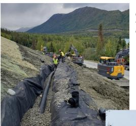
Crew works to install the underdrain systems on the slope.
