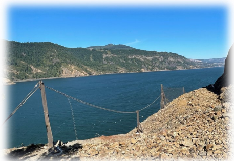
Left & Right: Hanging mesh rockfall protection fence on West Side
