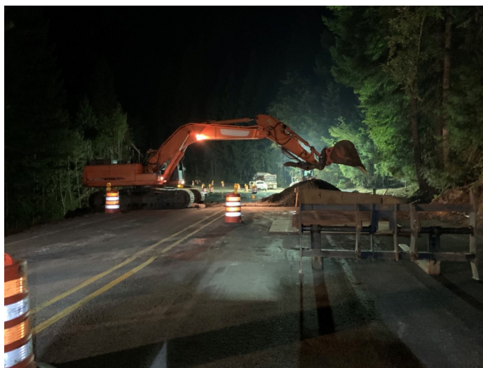
Photo left: Shows excavation of culvert at MP 56. All images Source: FHWA
