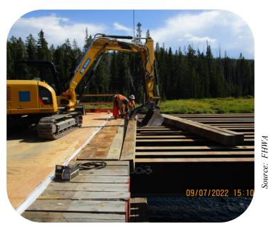
Steel girders and timber decking placed on temporary work bridge.
