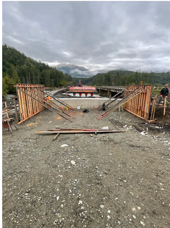
Left: Abutment 1 wingwalls being formed.
