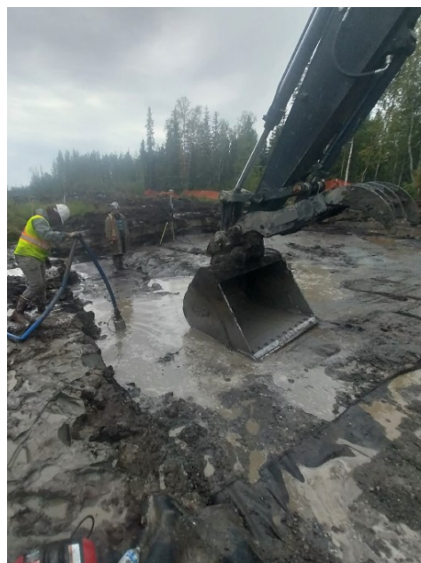
Left: Subexcavation on Lathrop St.
