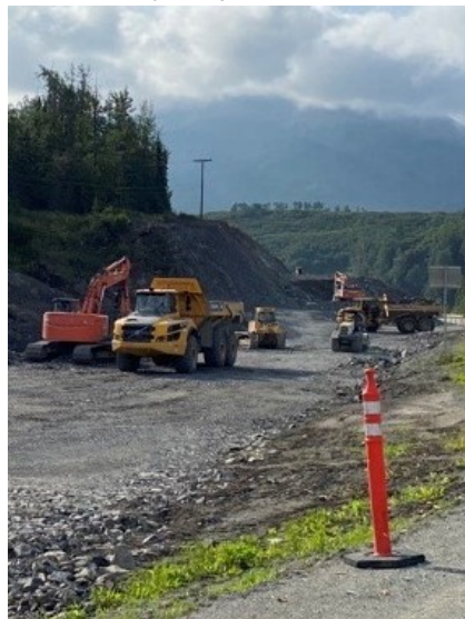
Left: Placing roadway embankment.
