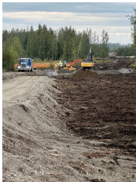
Left: 4-foot subexcavation on Northlake Lane at Lathrop St.
