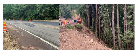
Photo left: Shows Finished temporary widening Photo Right shows clearing and grubbing down slope. All images Source: FHWA
