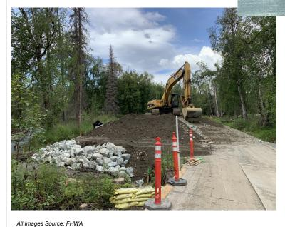
**Left:** Placement of Riprap around the South Fork Side Bridge abutment.
