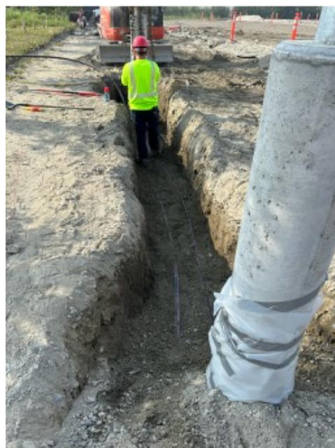
Left: Installing HBO posts and conduit at Motorized Boat Launch.
