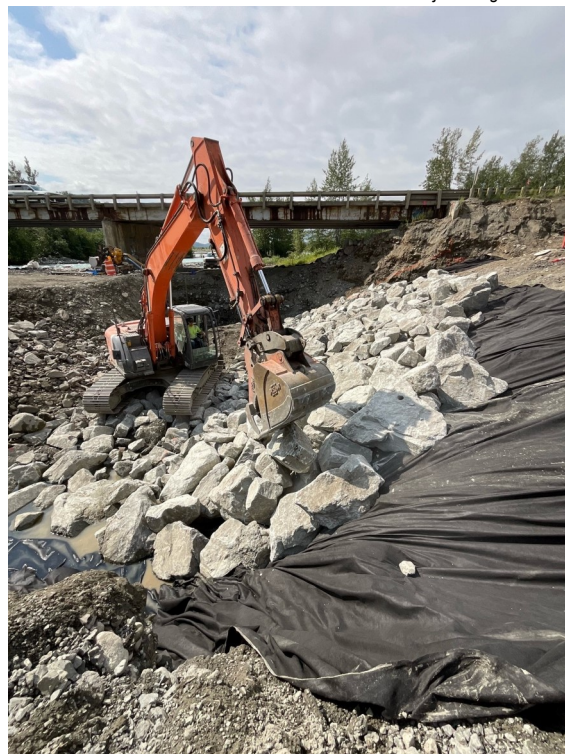
Left: Placing riprap.
