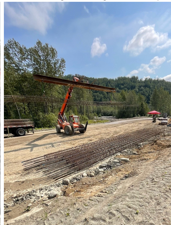
Right: Rebar cages for concrete pile.
