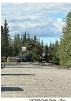
Left: Roadway aggregate being placed at the Motorized Boat Launch.
