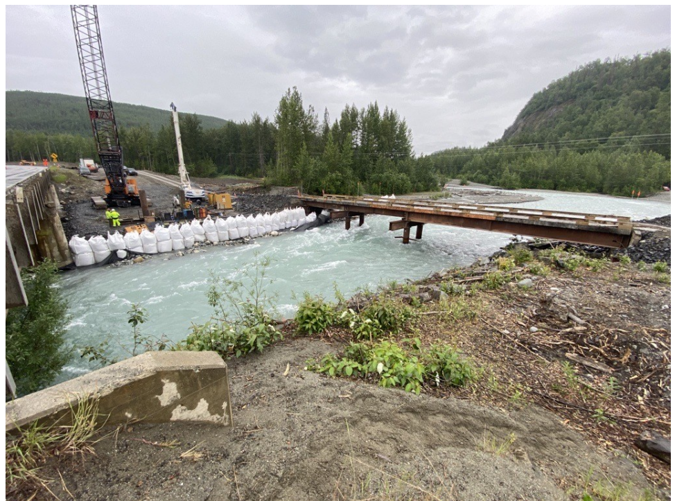
Photo: Temporary bridge, stream diversion sand bags, and piling driving equipment.
