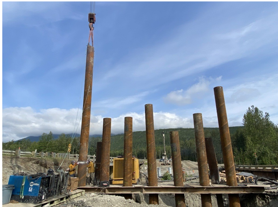
Photo: Welding pile at the south abutment.
