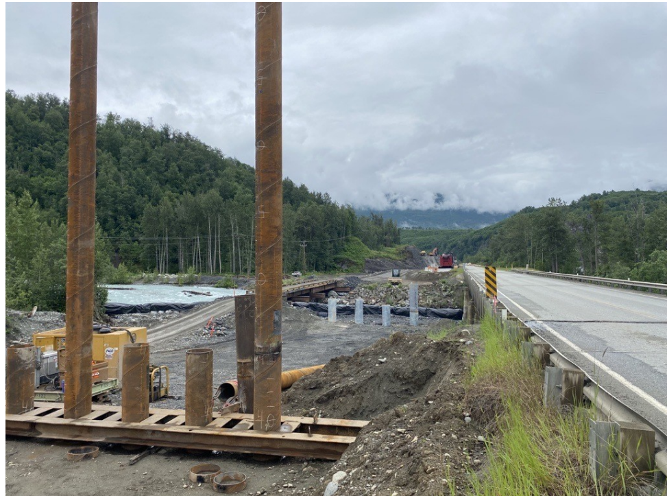
Photo: Pile driving at the north abutment.
