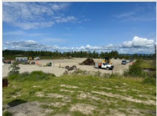
Below: Swim Beach Parking Lot Expansion looking NW.
