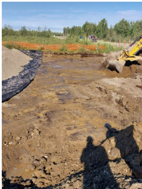
Left: Sub-excavation of the Swim Beach Expansion area.
