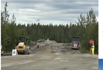
Left: Select Borrow being compacted over geotextile fabric on Lathrop St.
