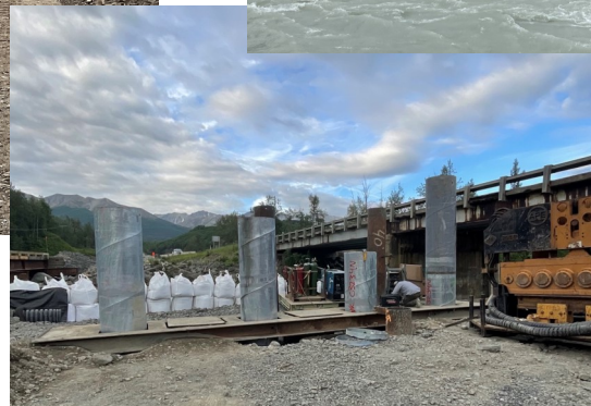
Above and Left: Galvanized piles at Pier 2.
