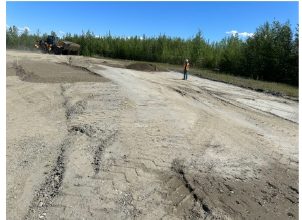
Above: Subbase being placed at the Motorized Boat Launch.
