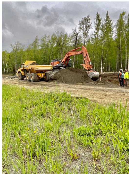
Above: Roadway excavation
