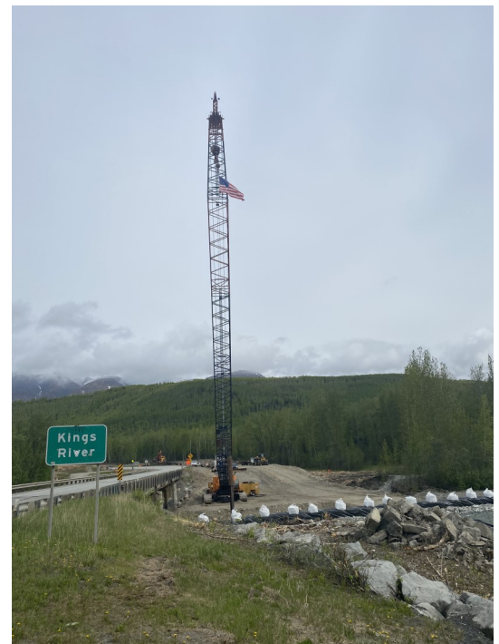
Above: Crane in place for pile driving
