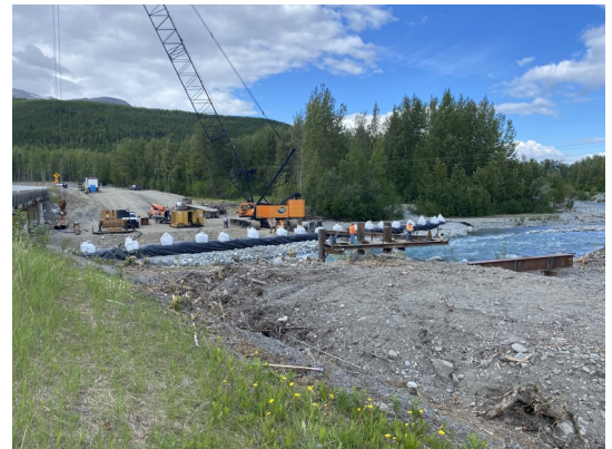
Above: Pile driving and stream diversion All Project Images Source: FHWA
