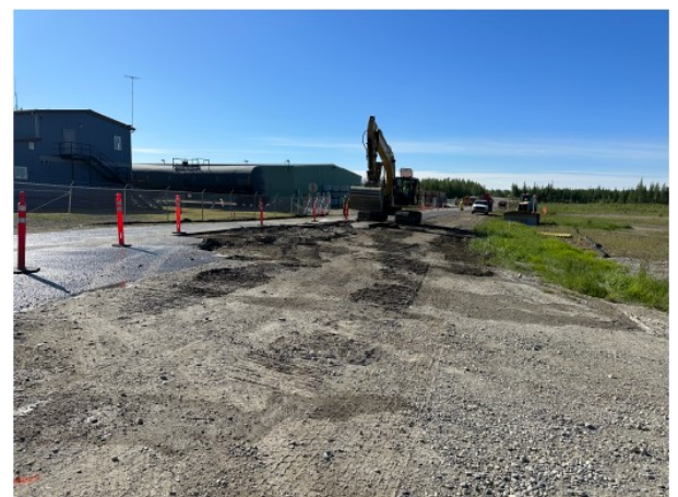
Above: Excavator is removing the old pavement on Lathrop Street.
