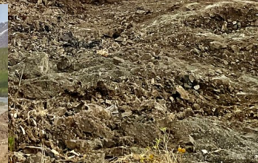
Above: Excavation operations
