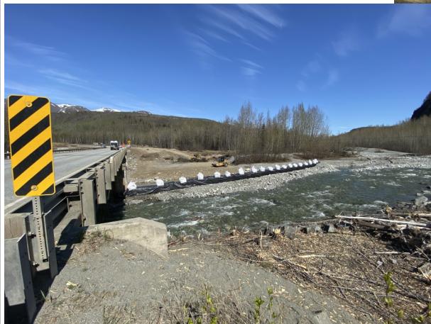
Left: Stream diversion in place.
