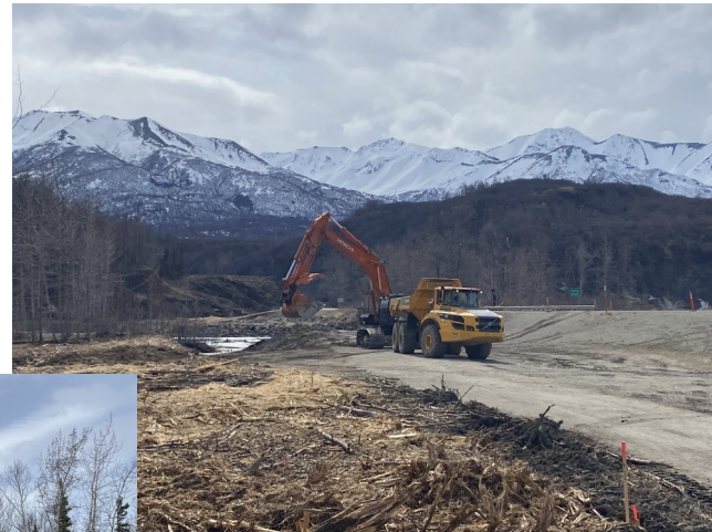
Right: Grubbing Operations
