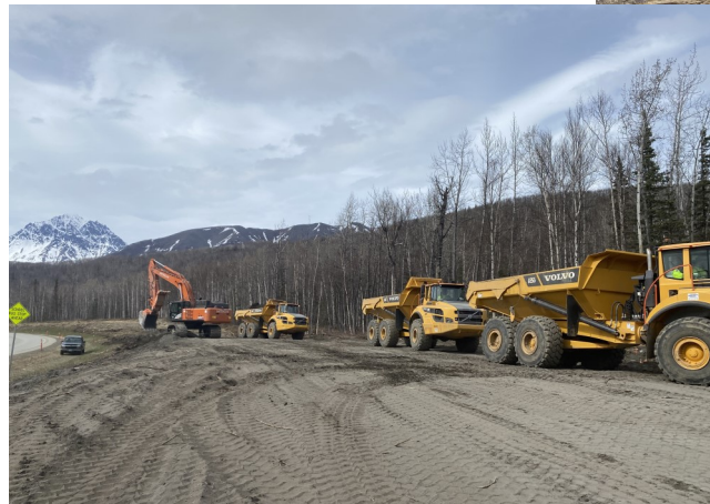
Left: Excavation operations
