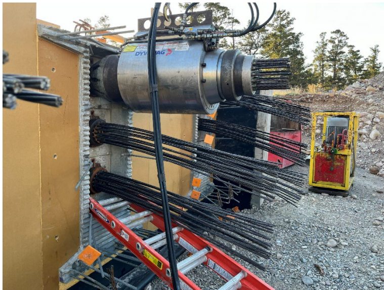
Post Tensioning Operations of the 3 Girder Lines
