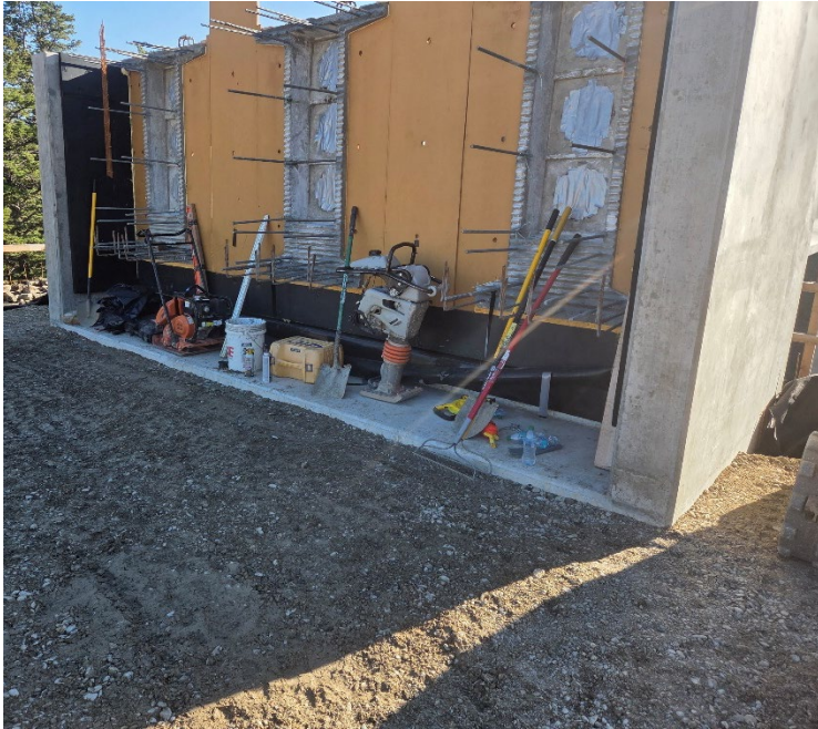
Abutment #4 on the East Side of Sun River
