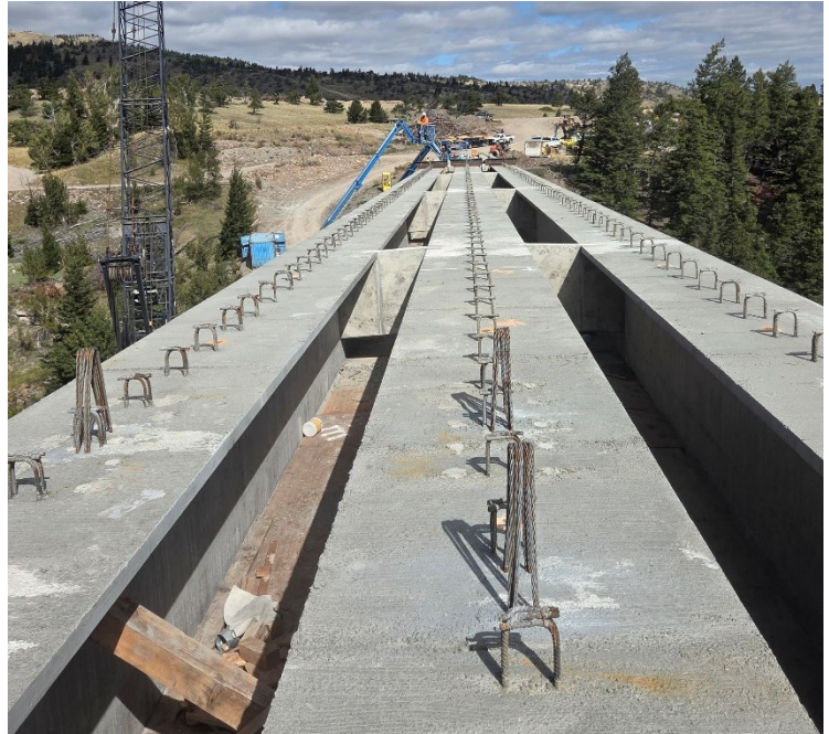
New Bridge Girders Looking from West to East over the Sun River
