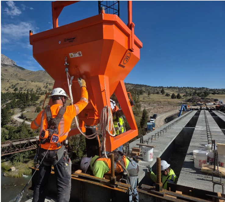
Placing Ultra High-Performance Concrete (UHPC) at 6 Girder Splice Locations
