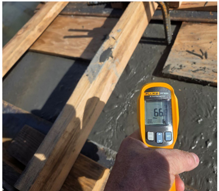
Crucial Temperature Measurements of UHPC Placement at Girder Splices
