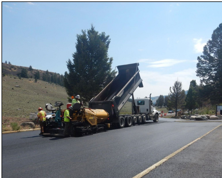
On Jul. 29, 2026, HK Contractors completed the top lift of asphalt paving on the Yellowstone River Bridge Trailhead Parking Lot.
