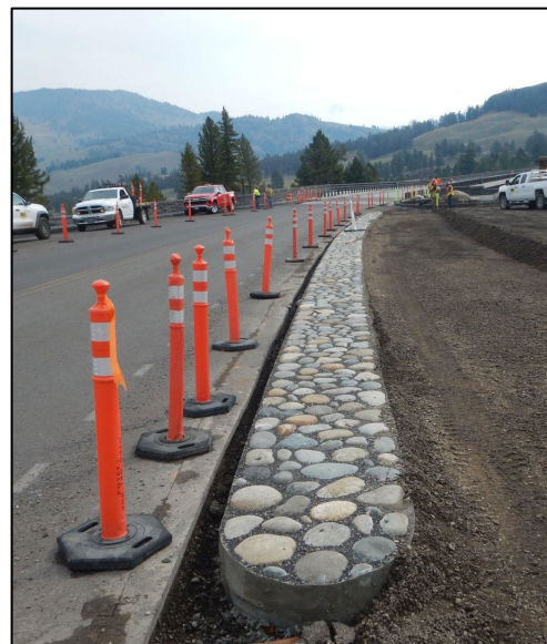
On Aug. 13, 2026, the decorative cobblestone median at the Bridge and Canyon Overlook Parking was completed.
