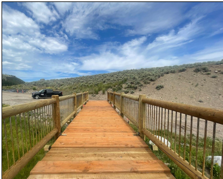
On Jul. 25, 2026, contractors finalized construction on the newly completed Equestrian Bridge, opening a safe pathway for horse riders and pedestrians.
