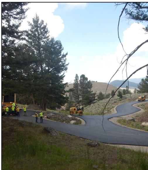
On Jul. 30, 2026, paving operations wrapped up the bottom lift asphalt layer on the Picnic Area Lower Loop.
