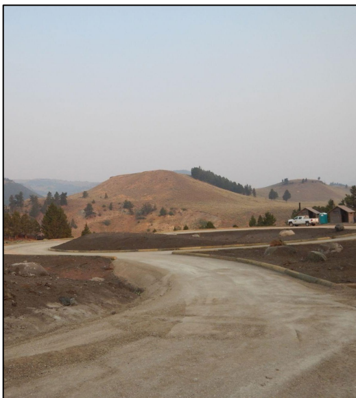
On Aug. 7, 2026, crews completed log curbing, topsoil placement, and aggregate base work at Wrecker Circle.
