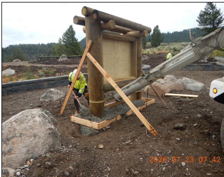
On July 23, Poteet Construction placed concrete to anchor the Informational Kiosk at the bridge/canyon overlook.
