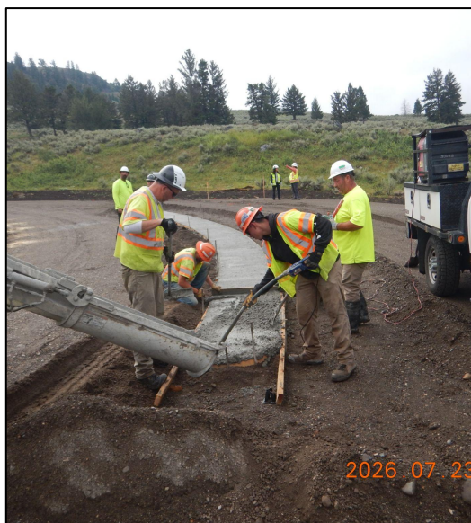
On July 23, Poteet Construction and HK Contractors placed concrete for the cobblestone median footing at Wrecker Circle.
