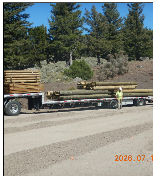
On July 16, log curb and Equestrian Bridge timbers were delivered to Wrecker Circle.
