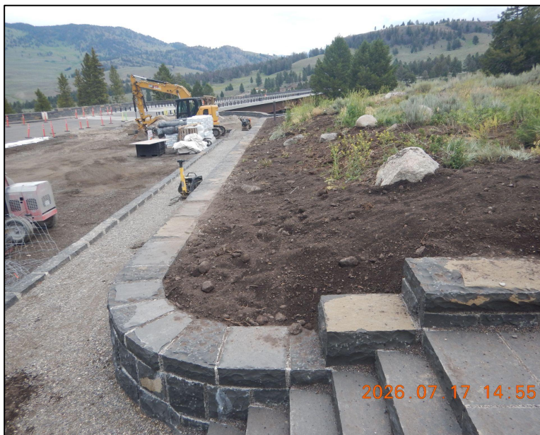
On July 17, the stone masonry wall and stairway at the bridge/canyon overlook is completed and backfilled.
