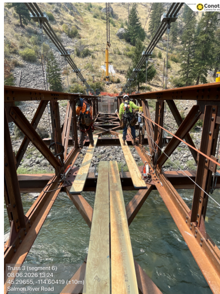
Splicing trusses together
