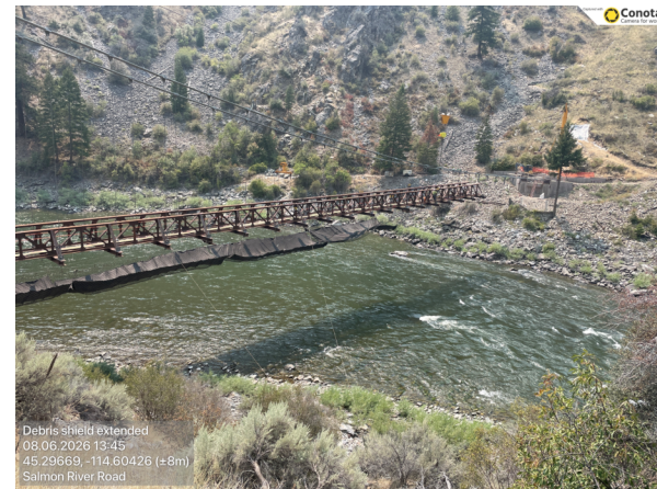
Steel structure installation
