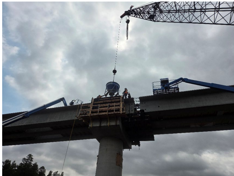
Pier #3 Cap Diaphragm Concrete Placement
