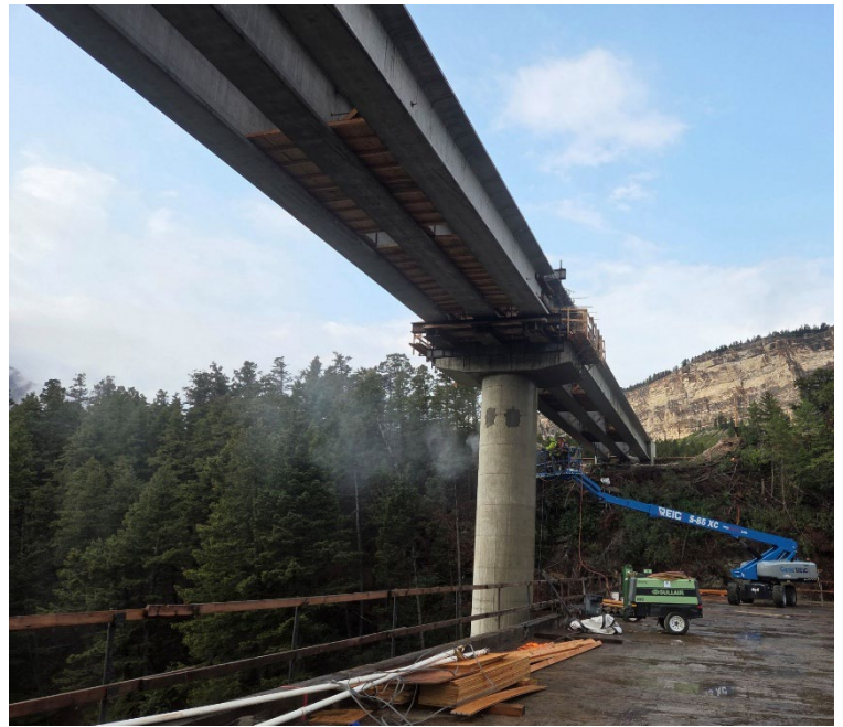
Pier #2 Concrete Finishing
