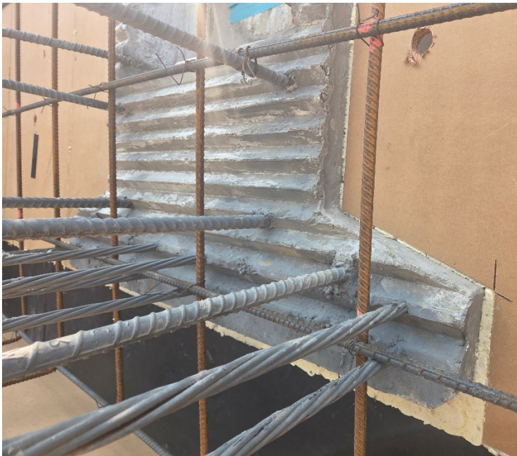
Abutment #4 End Diaphragm Formwork
