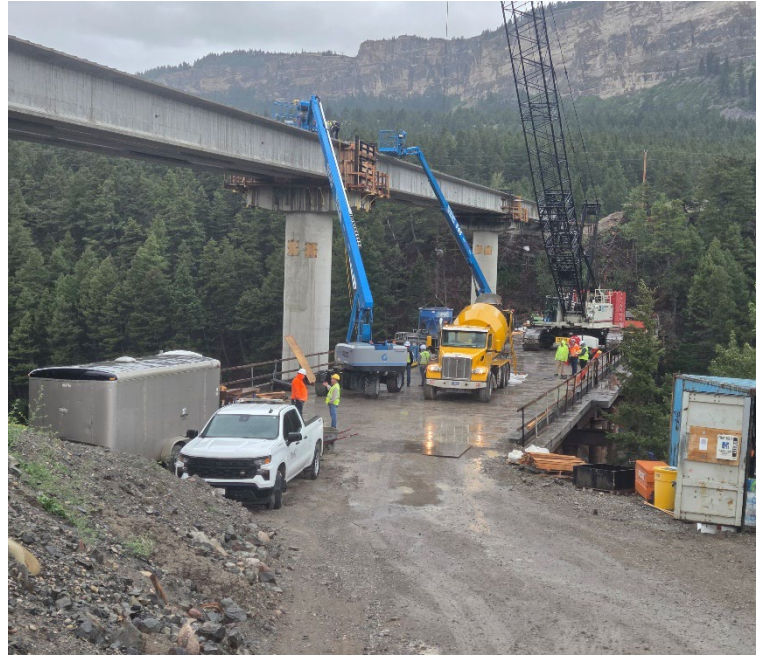
Pier #3 Cap Diaphragm Concrete Placement
