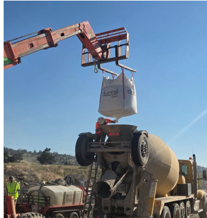
Mixing of UHPC for the Test Section
