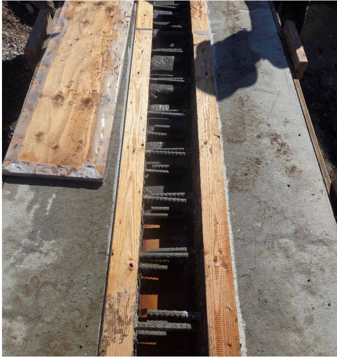
Ultra-High-Performance Concrete (UHPC) Test Section
