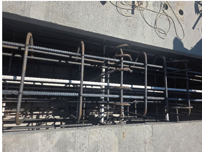
Pier #3 Girder Diaphragm Reinforcing Steel
