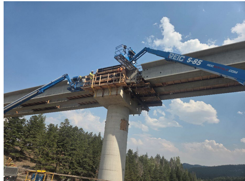
Installation of Pier #3 Cap Diaphragm
