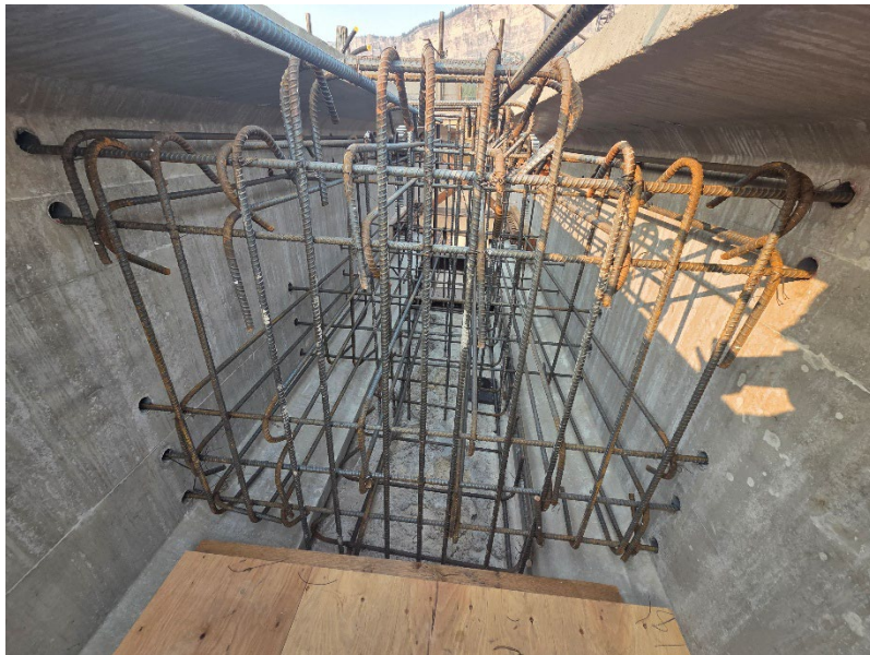
Intermediate Girder Diaphragm Rebar
