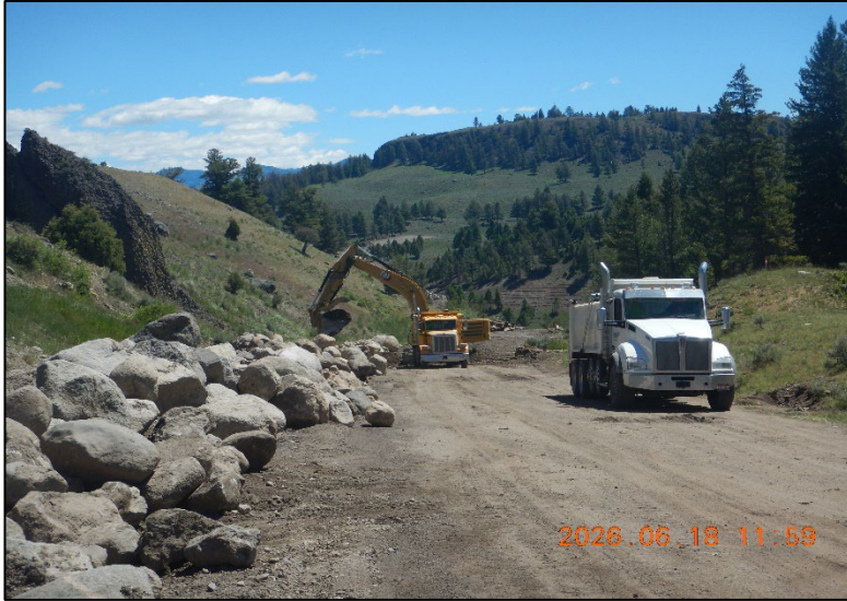
Lost Creek Restoration - Native boulders are stockpiled alongside the active work zone for upcoming stream channel restoration, stabilizing banks and creating healthy habitats.
