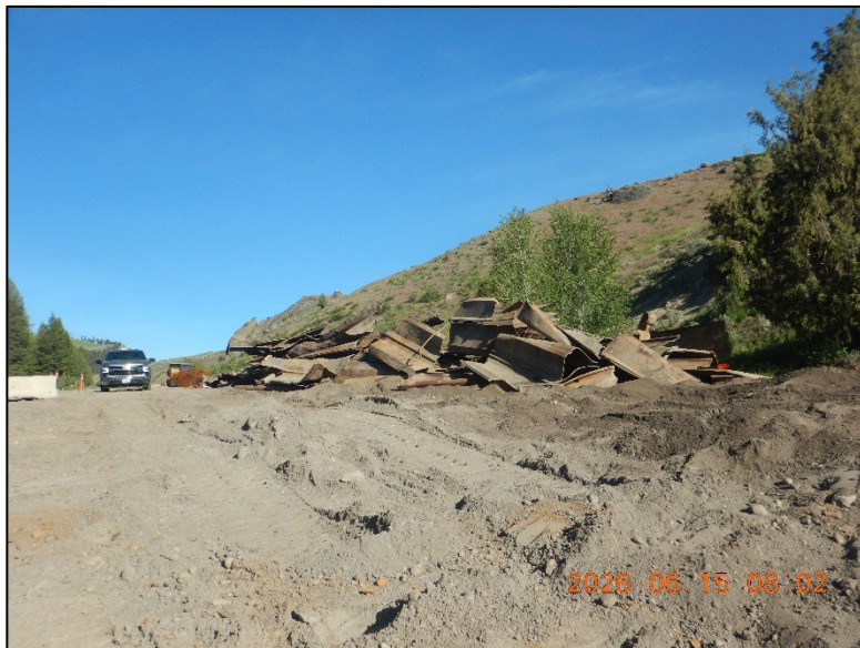
Pier #2 Progress – Temporary steel sheet-piling is extracted and staged for removal off-site. This structural removal clears the way for final grading into its post-construction state.
