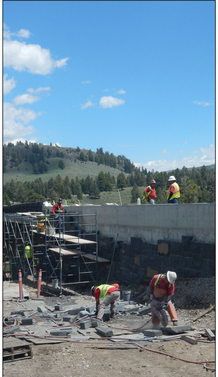
Wing-Wall Masonry – Crews with Guinett Masonry place native stone veneer along the outside face of wing-wall "A" to blend the new structure with the park's aesthetics.
