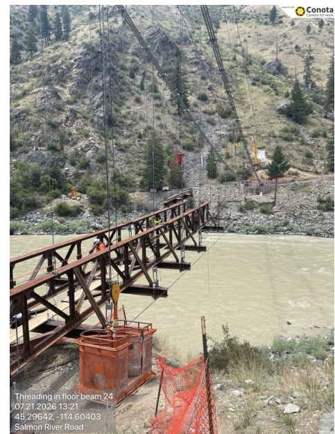
Steel structure installation
