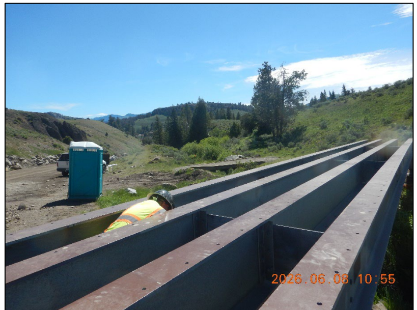
Construction crews install bridge girders at the Equestrian Bridge as work progresses on this key project component within Yellowstone National Park.
