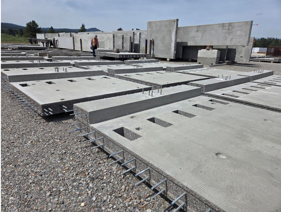
Completed Precast Concrete Deck Panels at Knife River Fabrication Yard in Spokane, WA.
