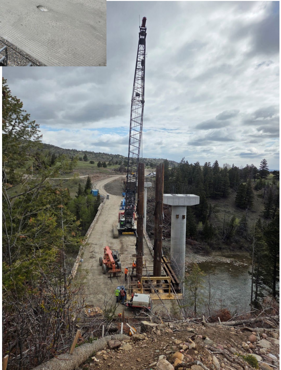
Crews Installing the Girder Launching Tower on the West Side of the River in Preparation of Girder Placement at the End of May.
