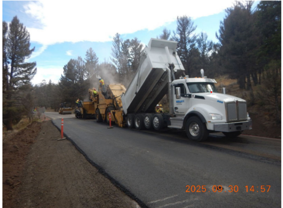
Paving at Northeast Project
