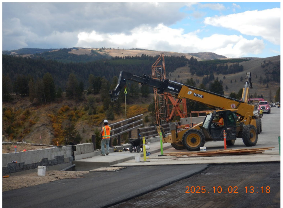
Installation of Bridge Railing Panel
