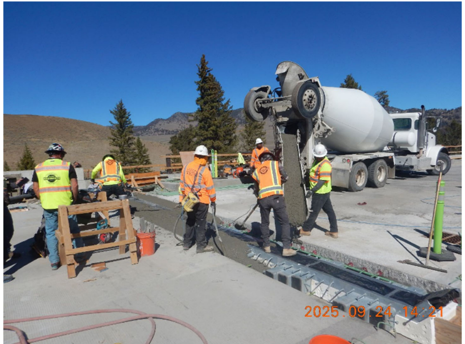
Installing Abutment 2 Expansion Joint
