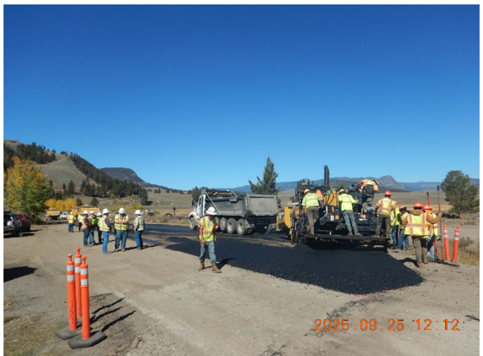
First Day of Asphalt Paving, Tower Row Parking Lot
