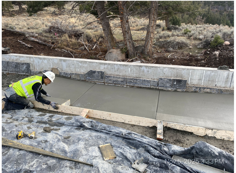
Completing Sidewalk and Pedestrian Ramp
