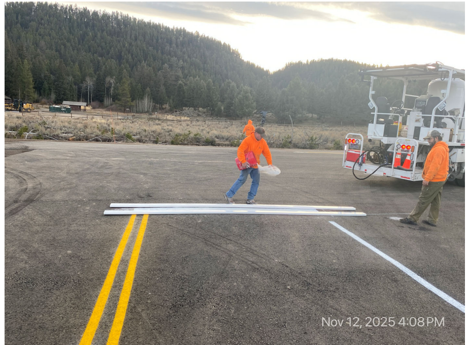
Worker applies reflective beads to freshly painted stop bar.
